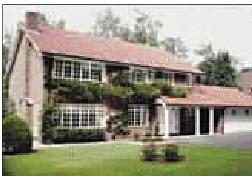
Left: A roof before getting the Moss Rid treatment, and (right) afterwards.
